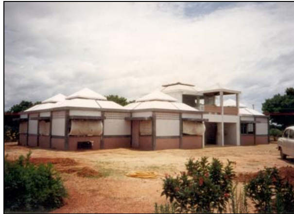
New Building in the Industrial Zone
